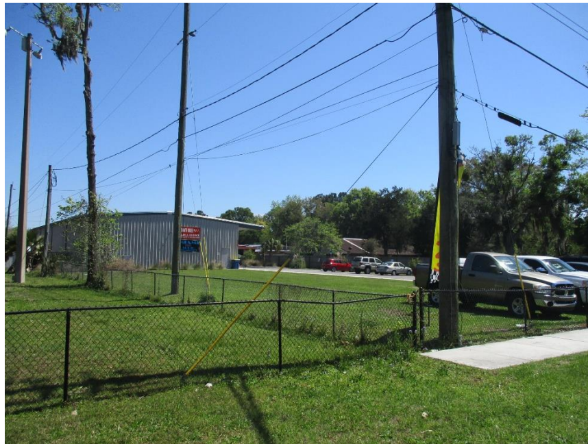
View of the neighboring property to the south of the subject property.
